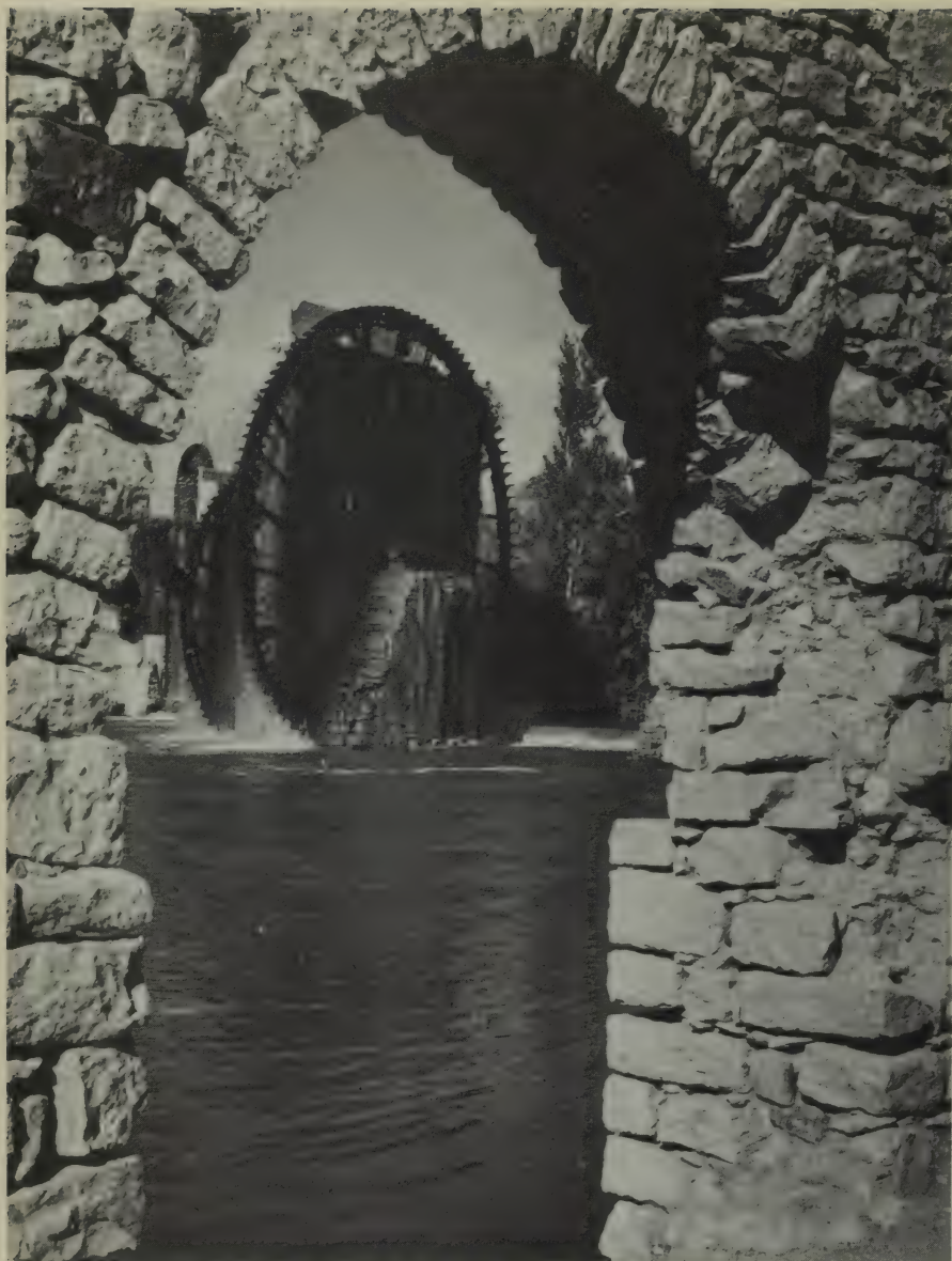
PLATE 14. The water wheels at Hama, on the Orontes River in Syria. The most famous existing examples of the noria , the earliest machine in which water power was used to perform work. The larger of the wheels shown here is some seventy feet in diameter. The aqueduct which receives the water from the top of the wheel and carries it away to irrigate the fields is of Roman construction. (Photograph by courtesy of the Syrian Ministry for Foreign Affairs)
